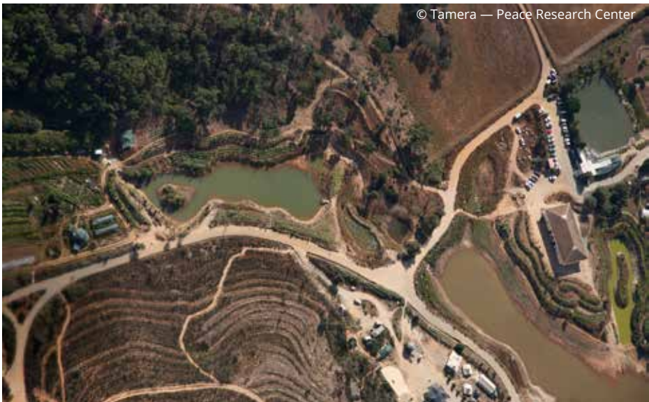
Aerial photo of the valley garden area after construction of the lakes was completed.
