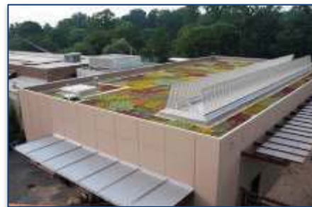
National Zoo: Elephant Trails, Green roof and operable skylights for natural daylight and ventilation on the completed barn
