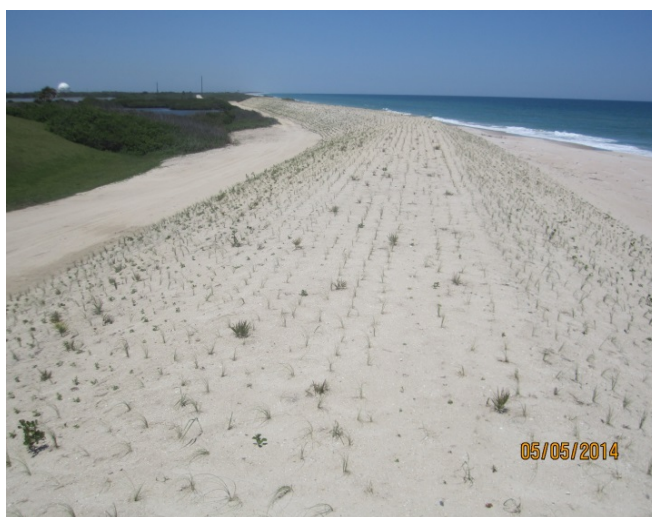
Dune repair at Kennedy Space Center
