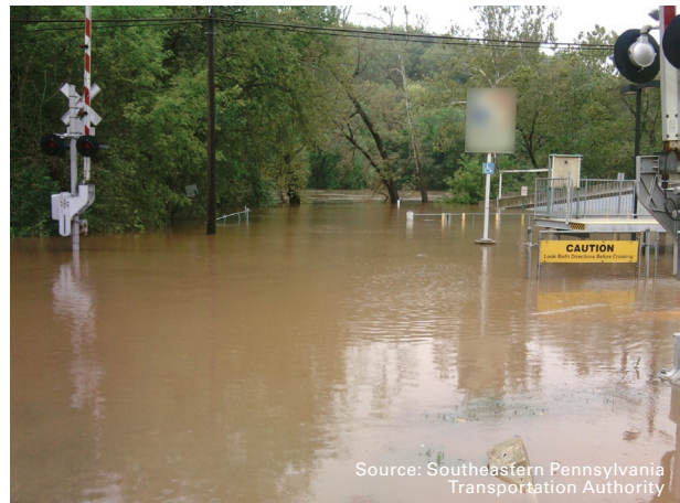
Figure 14. Photo. Flooding at Spring Mill Station on Southeastern Pennsylvania Transportation Authority's Manayunk/Norristown Regional Rail Line in Philadelphia.
